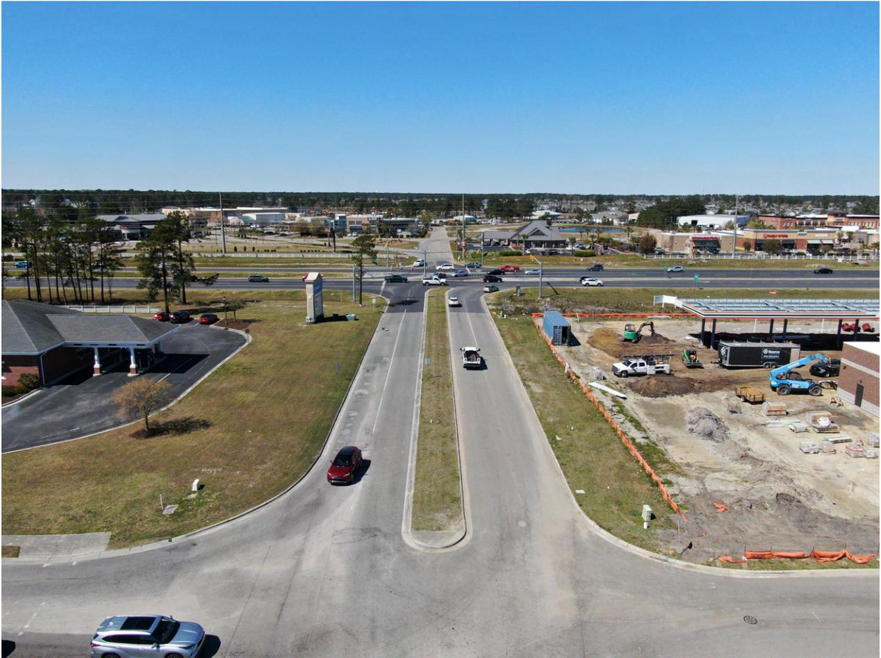
The scope of the project includes installation of a single-lane teardrop roundabout, new sidewalk connections to commercial developments, pedestrian improvements, resurfacing of Ocean Gate Plaza, and drainage improvements. The project will help to alleviate traffic in the surrounding commercial areas.
