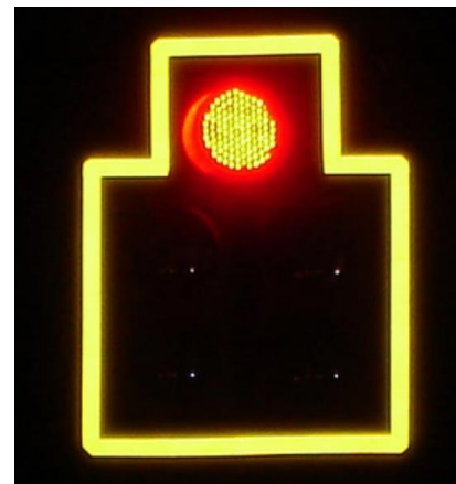
Signal Backplates with Retroreflective Borders (Source: FDOT)
