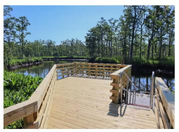
The Public Works Department completed the replacement of the former boardwalk at Cypress Cove Park. The replacement occurred on the deteriorating wood on the boardwalk, handrails, and the observation deck, providing residents with a safer deck to access and observe Mill Creek.
